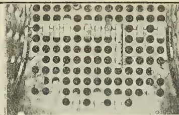
Fig. 5 New section of sheet ready for welding and riveting.
